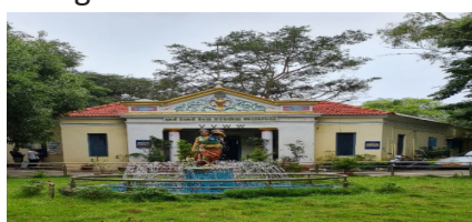
Vanivilas Water Works
