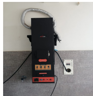
Sanitary napkin Incinerator
