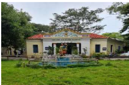
Vanivilas Water Works
