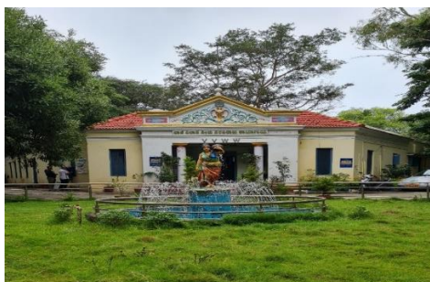
Vanivilas Water Works
