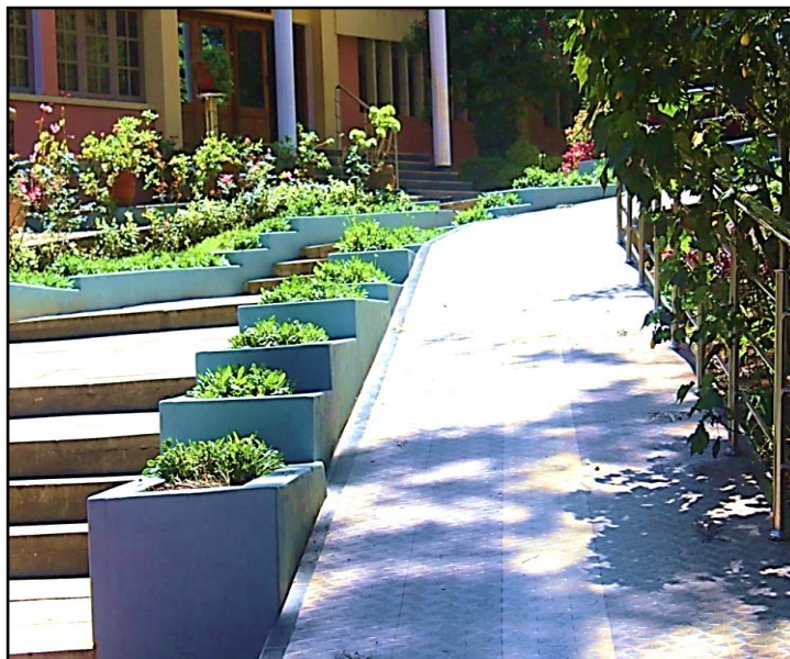
Ramp for Physical Disabled Students for Ease Of Access
