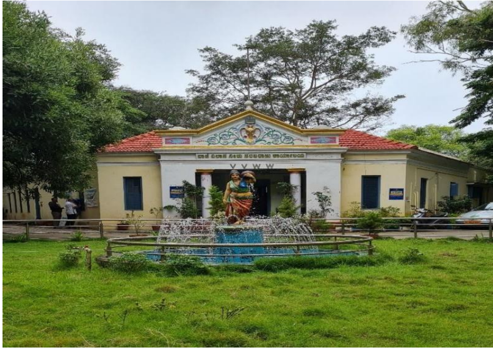
Vanivilas Water Works
