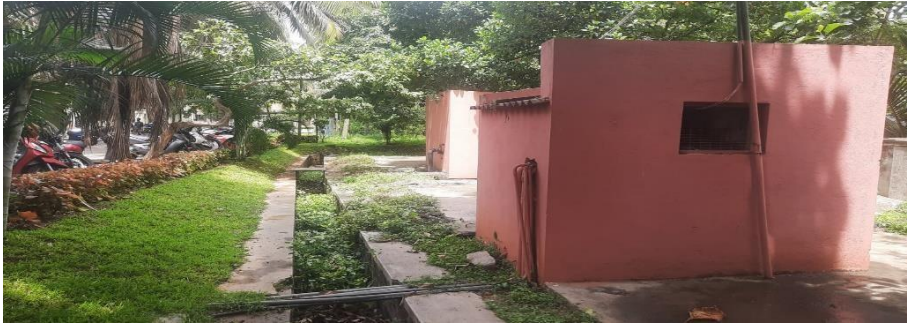
Waste water storage facility
