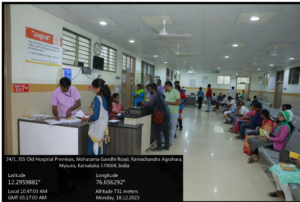
LED bulbs at JSS Hospital, Mysuru
