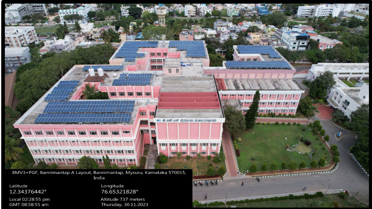
Rooftop Solar panel – JSS Medical College, JSS AHER, Mysuru
