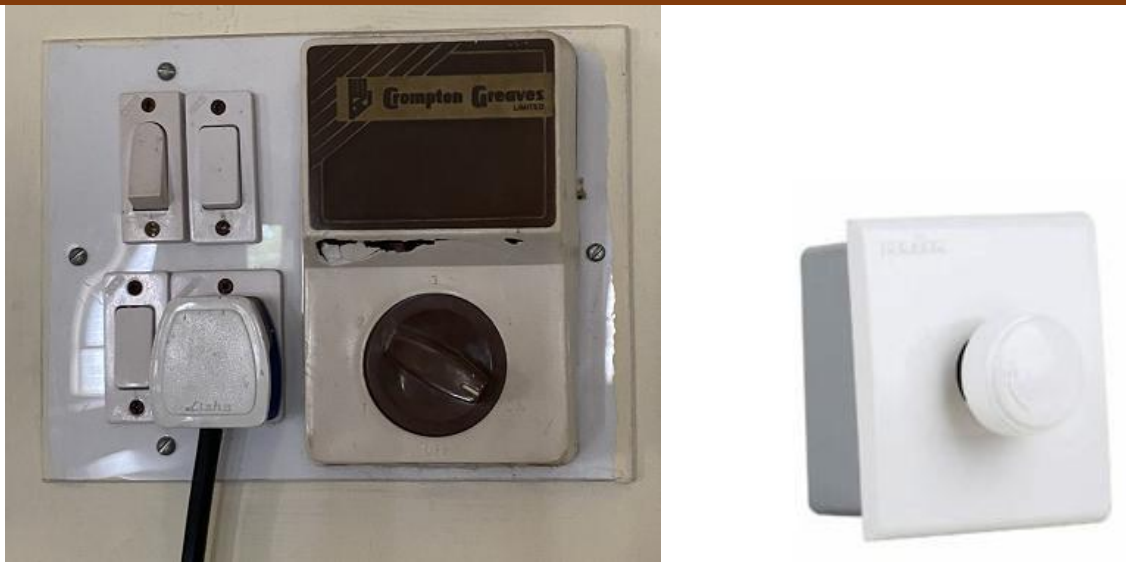
Fig 35: Old Rheostat type Fan Regulator in the campus & Proposed Electronic Regulator
