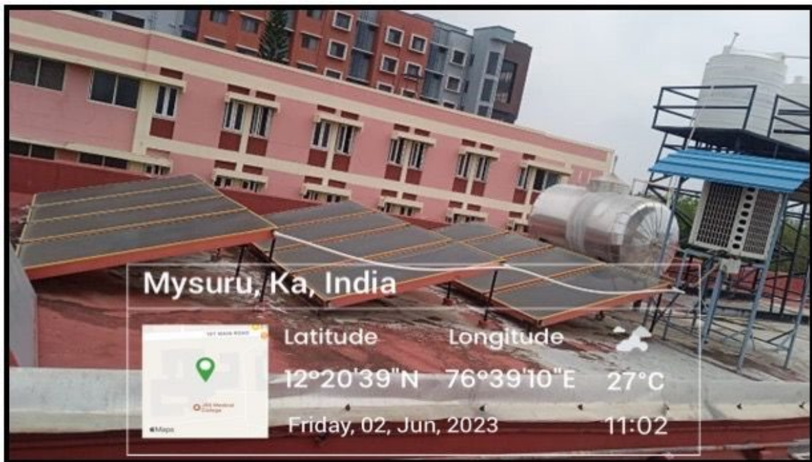
Solar energy powered water heater at hostel block, JSS AHER, Mysuru
