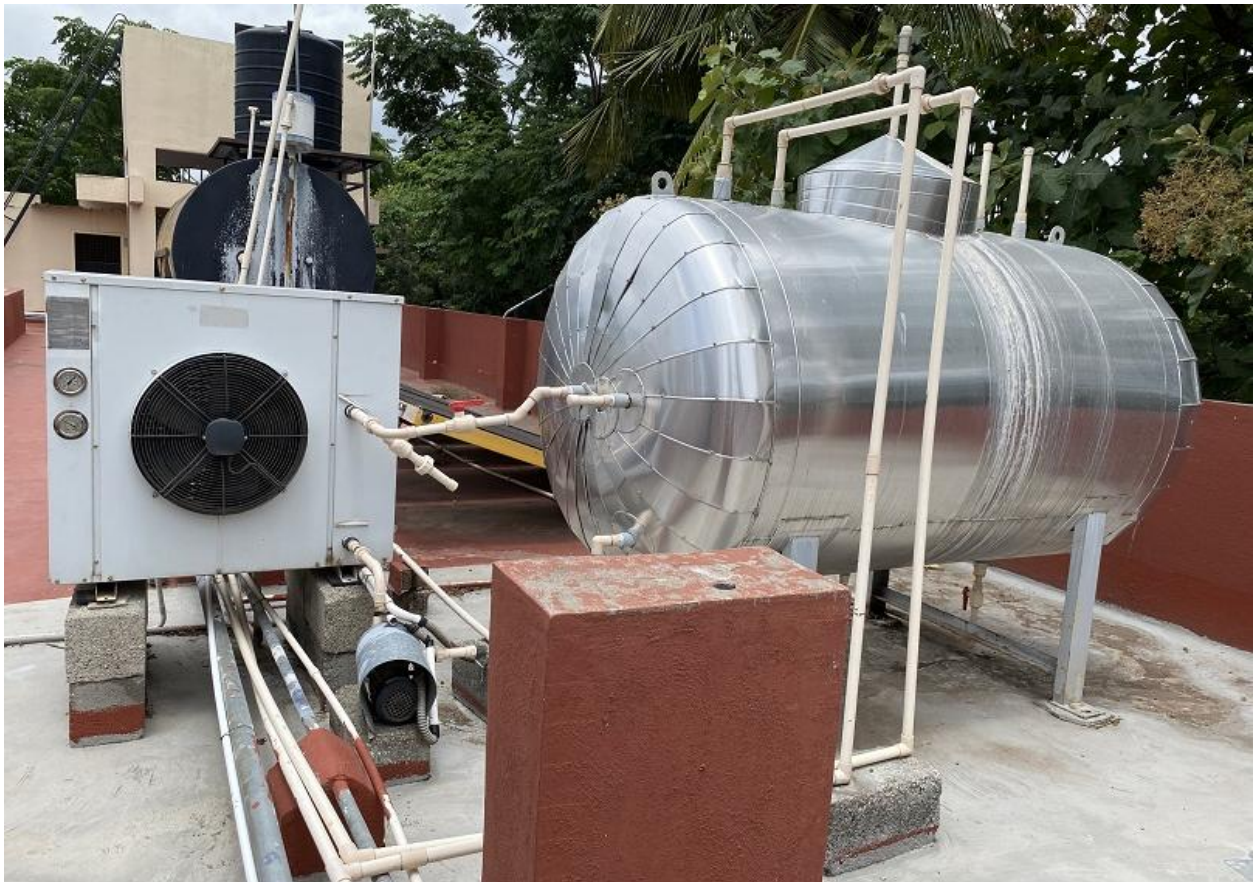
Fig 42: Existing Heat pump in Pharmacy Hostel
