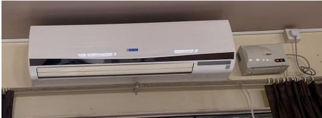
Fig 37: Old Non-inverter AC in the campus
