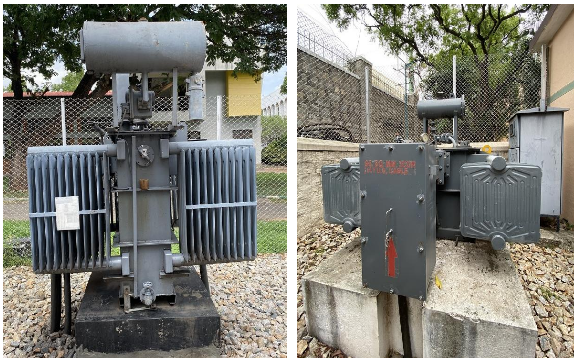
Fig 4: Transformers installed for incoming supply in Medical College and Pharmacy College
