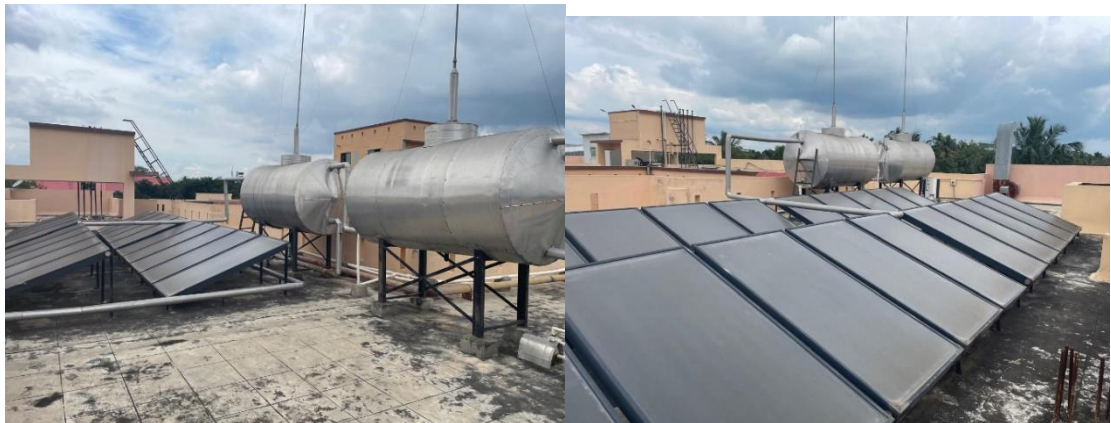
Hybrid solar water heater for cooking at JSSAHER
