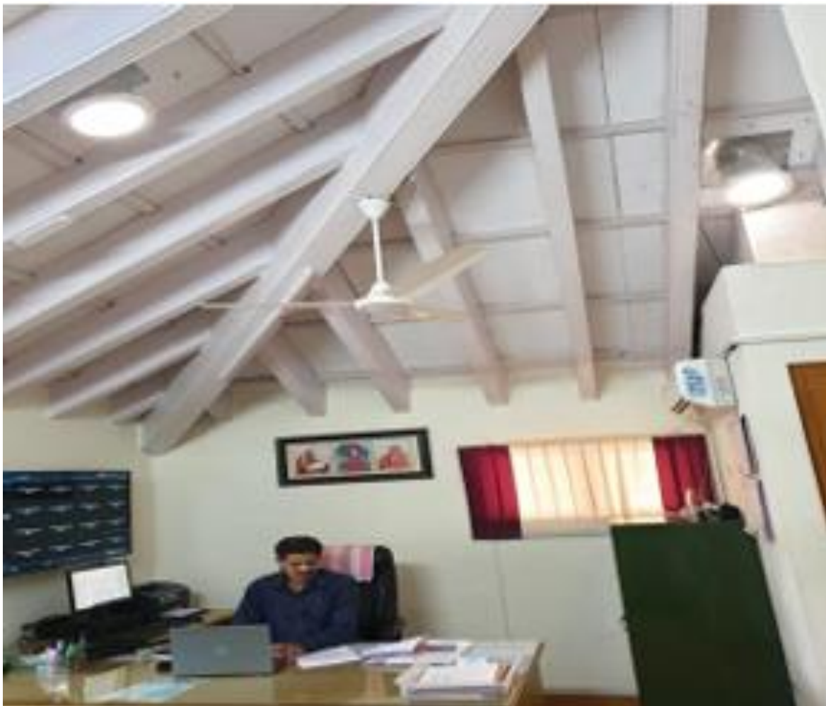
Natural light enhancer (Solar tube) for indoor lighting at JSSAHER campus
