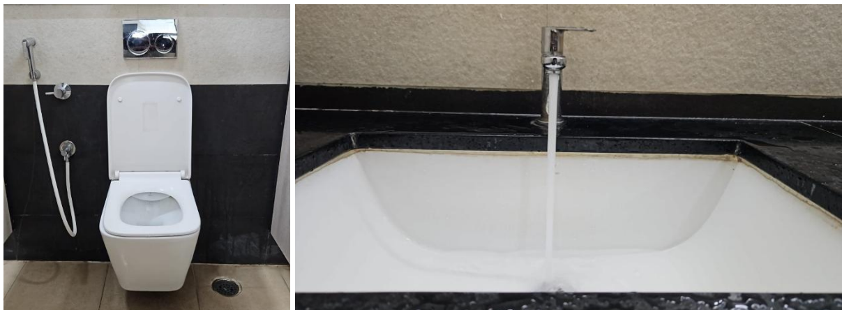
Installation of water-efficient fixtures and dual-flush toilets at JSS AHER Campus, Mysuru
