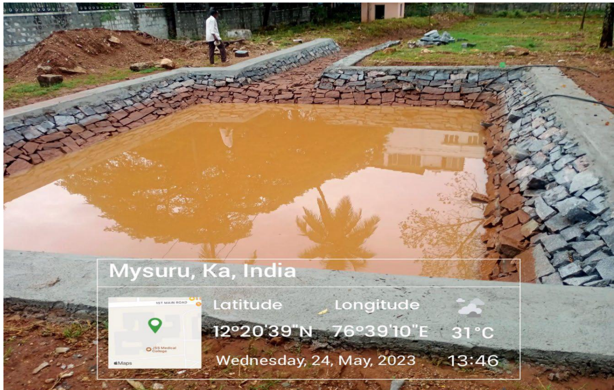
Collects and utilizes rainwater through recharging pits and ponds at JSSAHER, Mysuru
