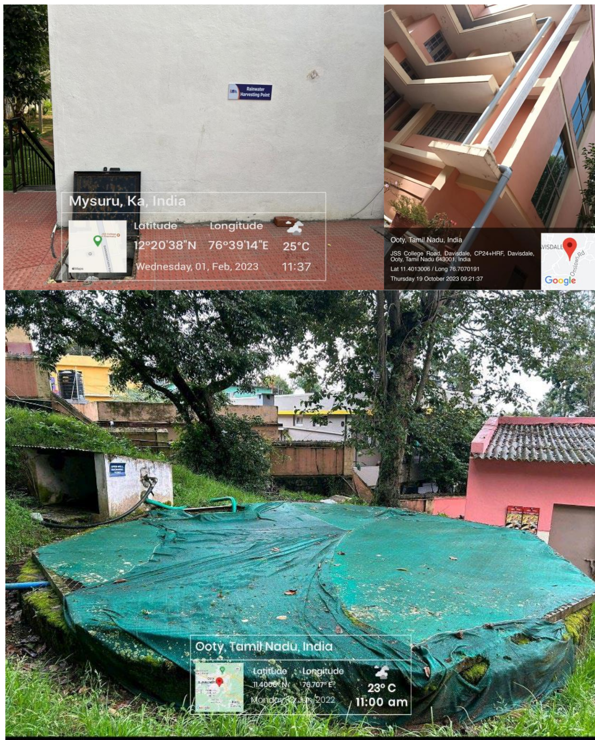
Rainwater harvesting system at JSS AHER Campus, Mysuru
