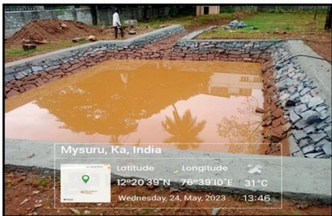
Rain water infiltration point at Hostel Block, JSS AHER, Mysuru
