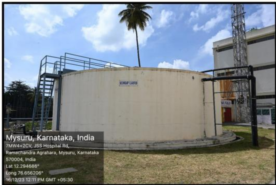
Secondary clarifier unit of water at JSS Hospital, JSS AHER, Mysuru
