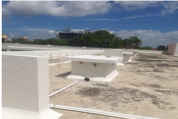
RAINWATER HARVESTING COLLECTION (SUMP)
