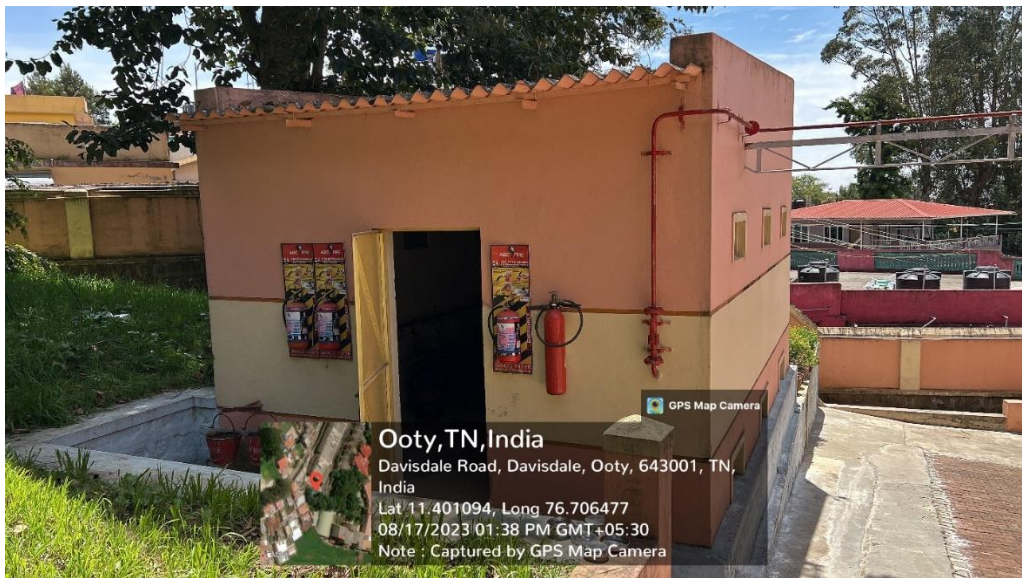
Safety measures taken at LPG cylinder storage area
