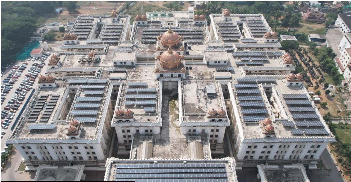
Solar panels are installed in the campuses of JSS Medical college and Hospital roof tops. The power generated through this is supplied to the grid.
