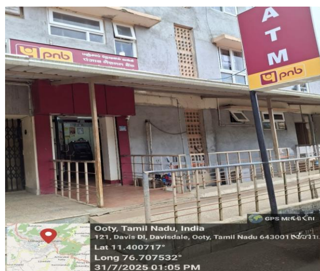
Picture represents the ATM Facility.
